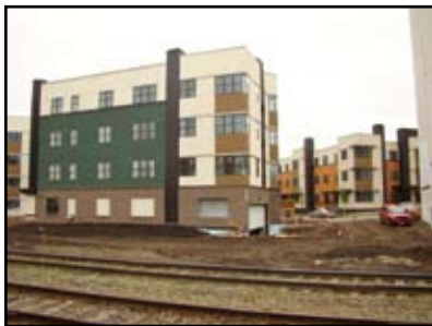
Phase II in the foreground with Phase I in the background. The Bunge Grain Elevator sits to the right.
