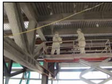
Mulcahy crew fireproofing the underside of the stadium deck.
